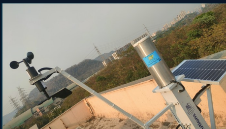
WIND SENSOR BOOM - CLOSE-UP
